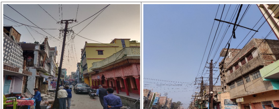
Non-execution of Ariel bunch cable in densely populated areas of Jamalpur and Lakhisarai
